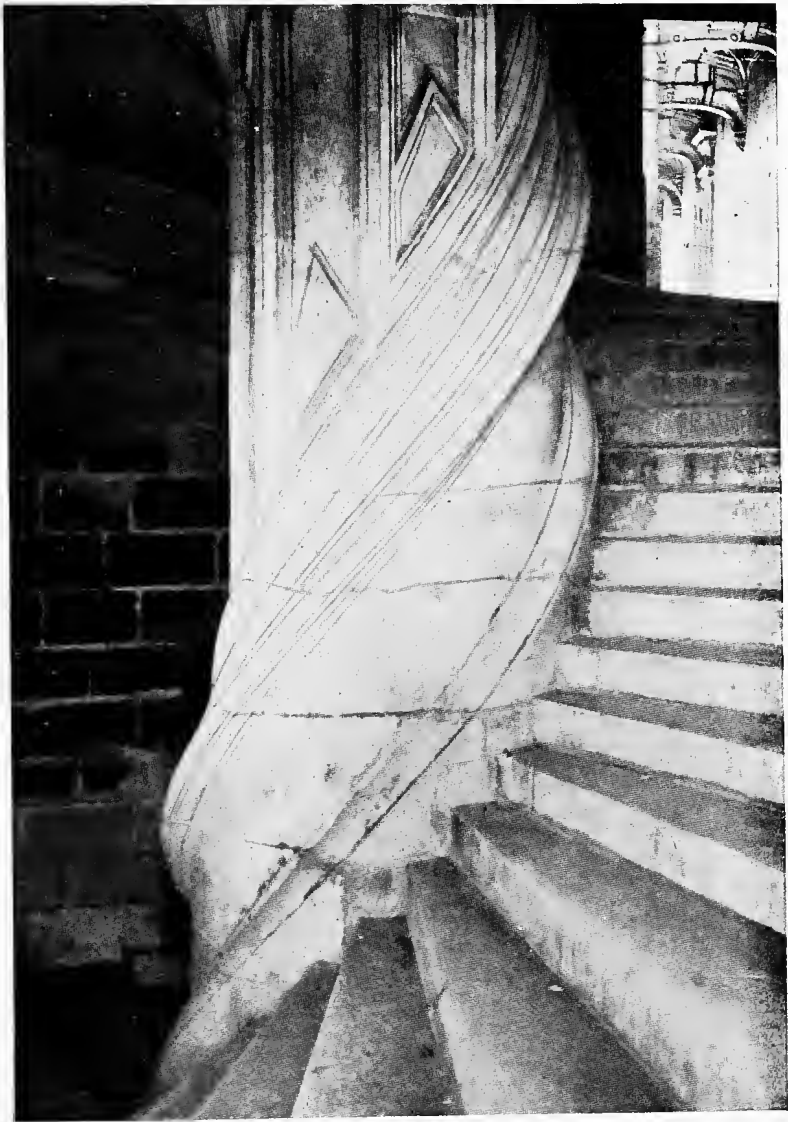
FIG. 347.—THE STRAIGHT STEPS OF AN ORDINARY RIGHT-HAND SPIRAL STAIRCASE IN A FRENCH RENAISSANCE CHÂTEAU.
