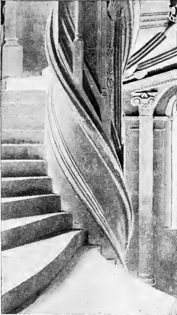
FIG. 346.—THE CURVED LINE OF THE STEPS IN THE OPEN STAIRCASE AT BLOIS.
