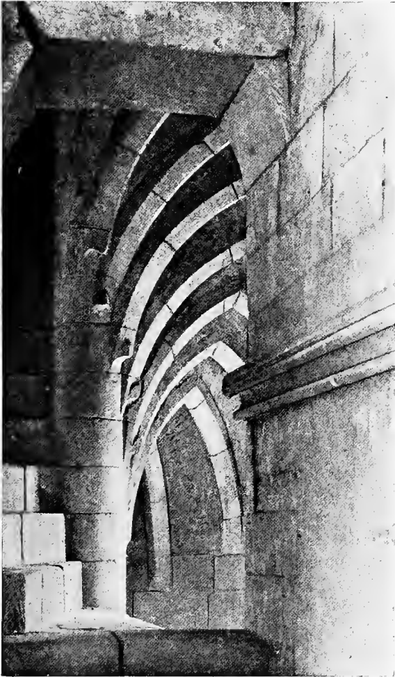
FIG. 321.—SPIRAL STAIR IN THE S.W. TURRET OF LINCOLN CATHEDRAL. (From a photograph by F. H. Evans.)
