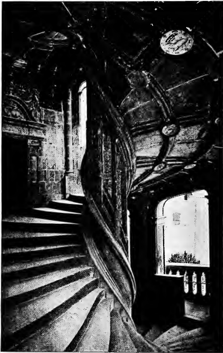
FIG. 343.—INSIDE OF THE OPEN STAIRCASE AT BLOIS, SHOWING THE SPIRAL LINES CARVED ON THE CENTRAL COLUMN AND THE VAULTING.
