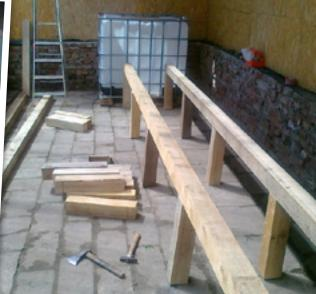
Heavy duty beams to support the growbed
