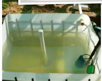
Sump tank with 6000lph pump and float switch
