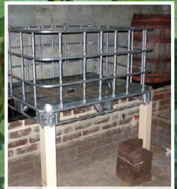
The metal base for the IBC is just deep enough that it can fit a 90 degree outflow pipe
