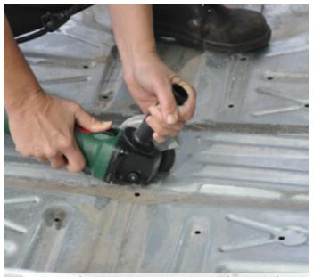
Cut the hole in the steel base large enough for the drain fittings
