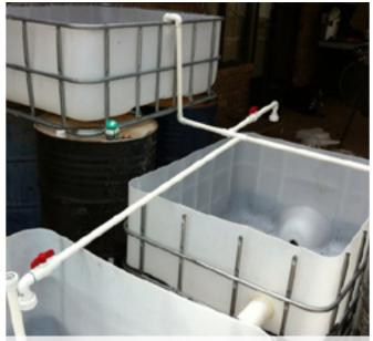
Irrigation line using 25mm pipe and ball valves
