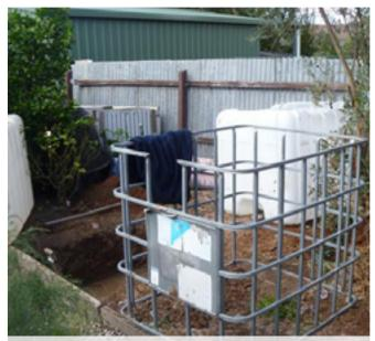
The steel base of the IBC cage is not required when burying
