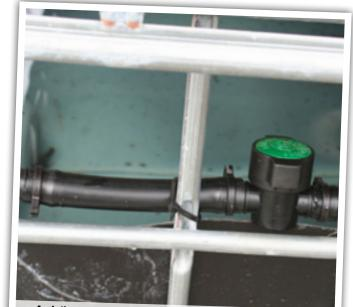
An inline tap allows for flow adjustment as water is pumped to growbed as well as to the surface of the fish tank providing additional aeration.
