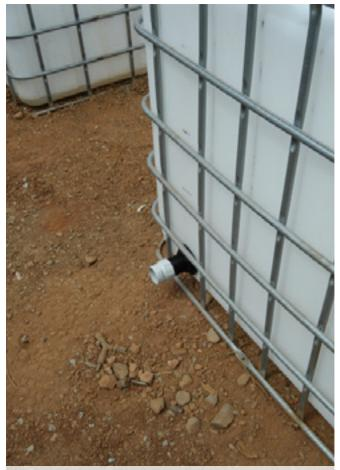
Tank fittings are one of the safest ways to plumb an IBC
