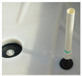
Standpipe using tank fitting, coupling and pvc pipe
