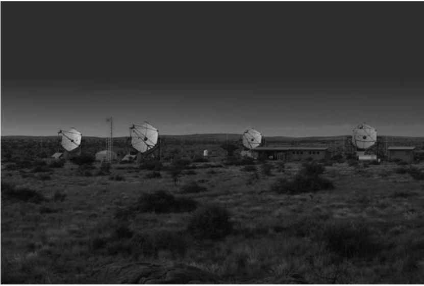
Fig. 11.7. The HESS gamma-ray telescope is located in the Khomas highlands of Namibia, a very dry region with excellent conditions for observing in the optical. Each of the 13-m telescopes consists of a collection of mirrors which bring the Cherenkov light to the focus. The multiple-telescope array allows the position of the gamma-ray source to be determined. Courtesy of the HESS collaboration.
