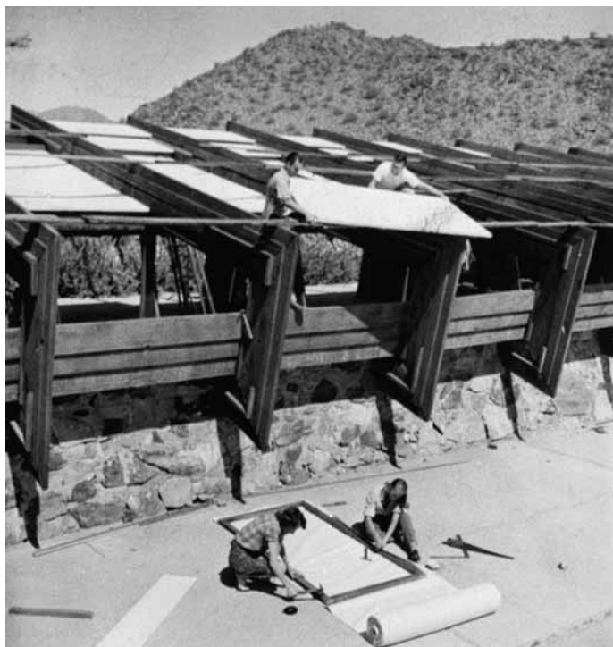
Taliesin West, Scottsdale, Arizona, 1937–9, apprentices putting canvas on roof frames.
