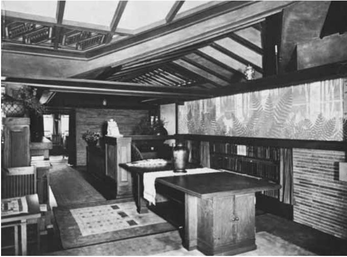
Interior of the Avery Coonley House, with hip ceiling. Riverside, Illinois, 1908.
