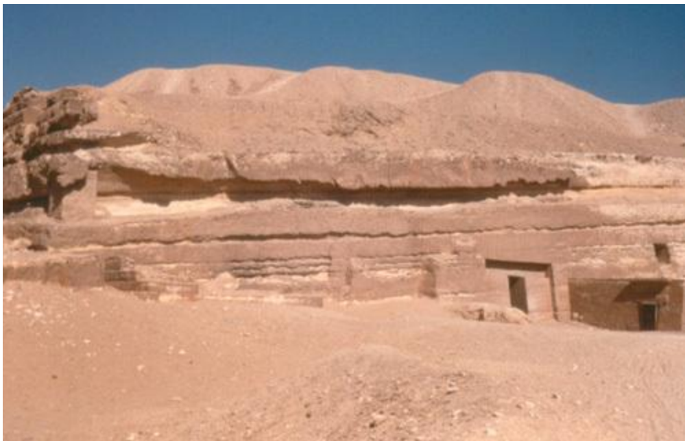
Plate 8. Wind-induced weathering and erosion on Old Kingdom tombs, Giza Plateau. Photograph taken by R. Schoch in the early 1990s.
