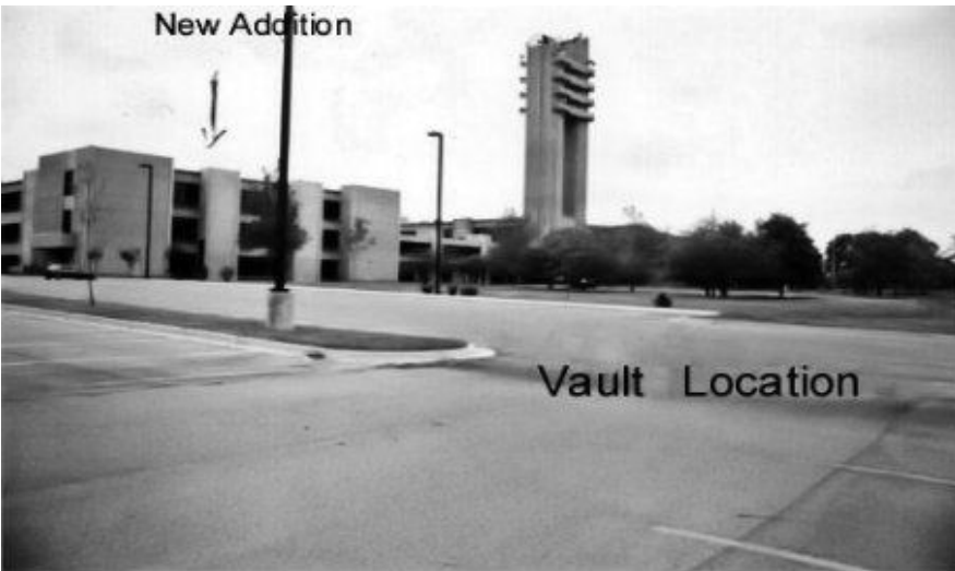
Figure 6: Parking lot paved over vault near building 620.
