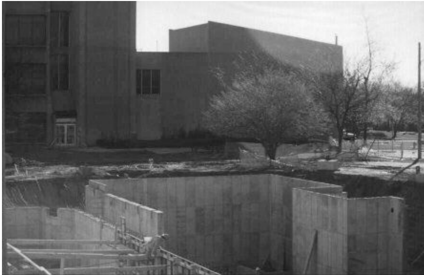
Figure 5: Building 620 expansion; northwest corner 1998.
