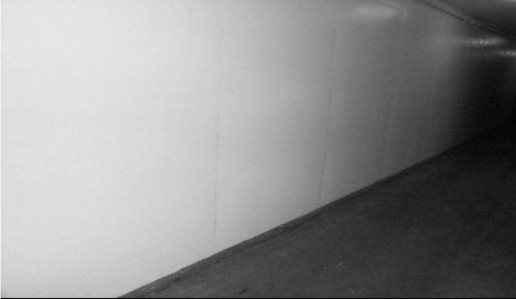
Figure 10: First basement west vault Bldg 620 showing newly walled up area.
