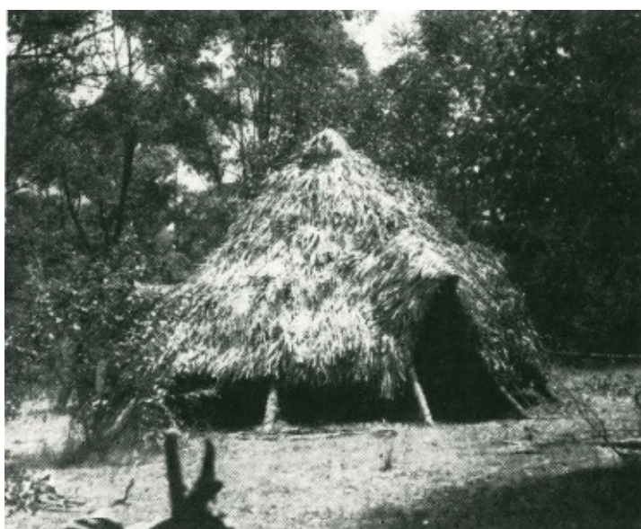
Circular hut 20 feet diameter at ground; no nails or man-made materials used in its construction. Time of erection, 12 to 18 man hours. Left half is thatched with palm leaves—right half thatched with eucalypt branches. Shortly after erection there was 4½ inches of rain in 75 minutes. The inside of the hut was completely dry after this terrific drenching.
