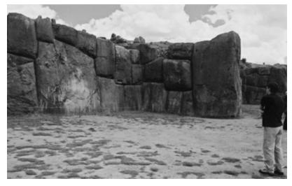
The site of Sacsayhuaman, located just above Cuzco, displays some of the largest and most extraordinary stones. The stones have several differently shaped sides, which somehow all fit perfectly together. This techniqe was necessary because of the severe earthquakes prevalent in the region. The Inca's construction technique has proven to withstand these quakes when no other buildings did.
