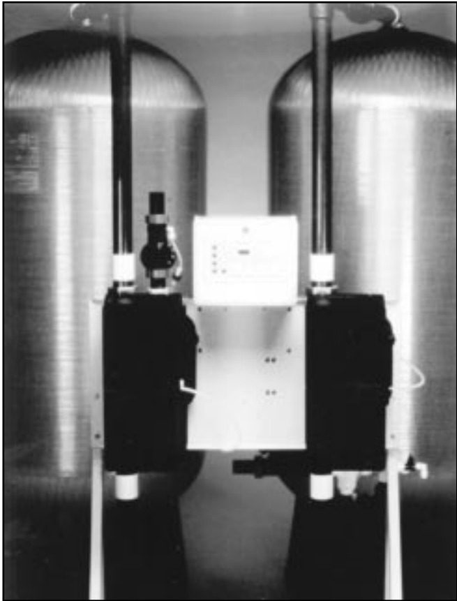
Figure 17 – Two-Bed Deionizer
