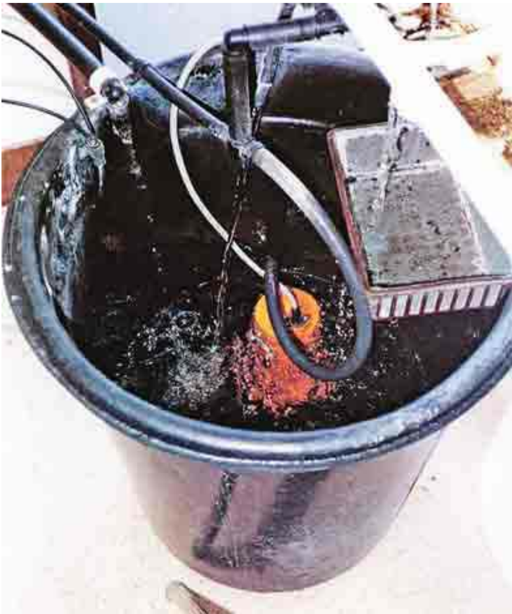
The drain tubes shown in the top right of the picture, in this system return the nutrient solution to the holding tank through a strainer to remove any unwanted material.
