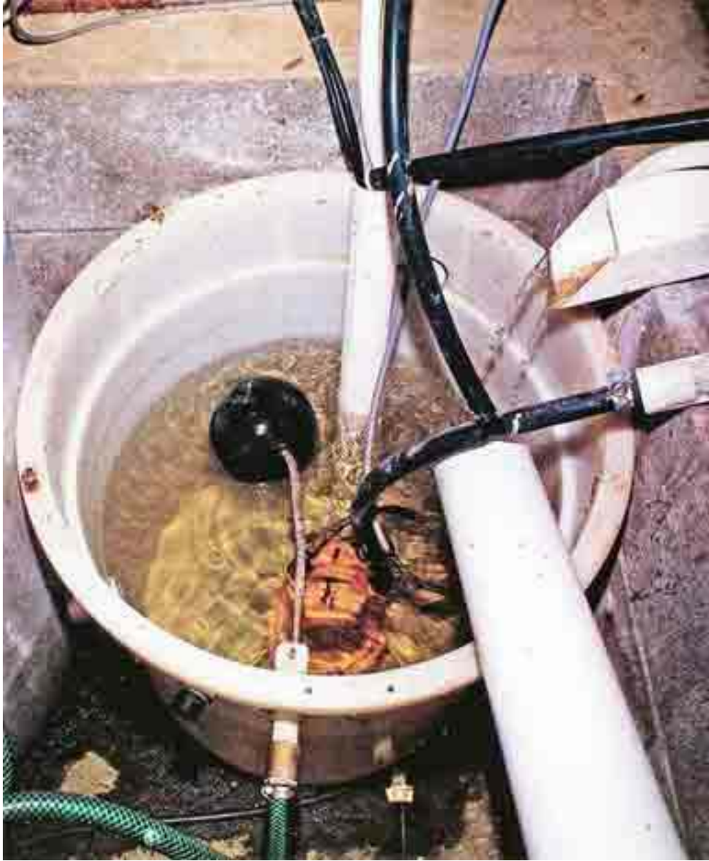
This white bucket is the holding tank for a home hydroponic system. The black float operates the water make up valve allowing extra water to flow into the tank when the level becomes too low. This float arm needs covering to stop the nutrient on metal contaminating the nutrient (See the obvious corrosion on the arm)
