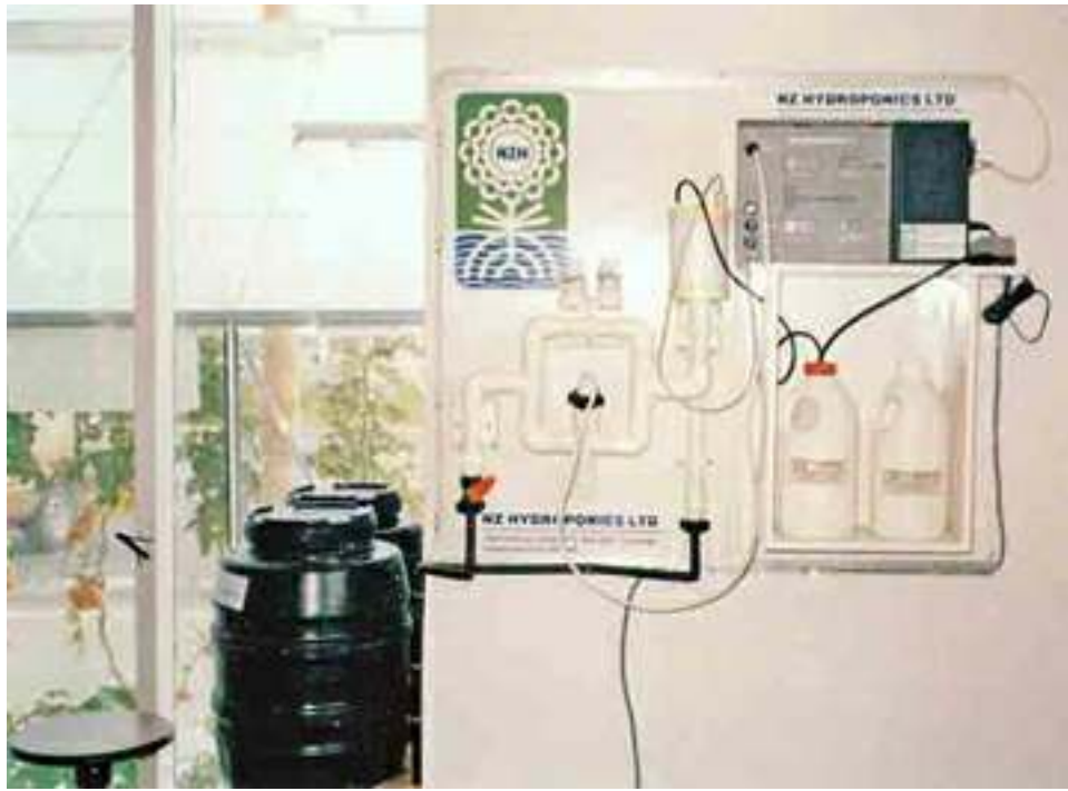
This installation shows an early 'Dosetronic' hydroponic controller mounted inside a building while controlling a hydroponic installation in the glasshouse outside. Note the two small PVC drums which hold the 'A' and 'B' nutrient stock solutions.
