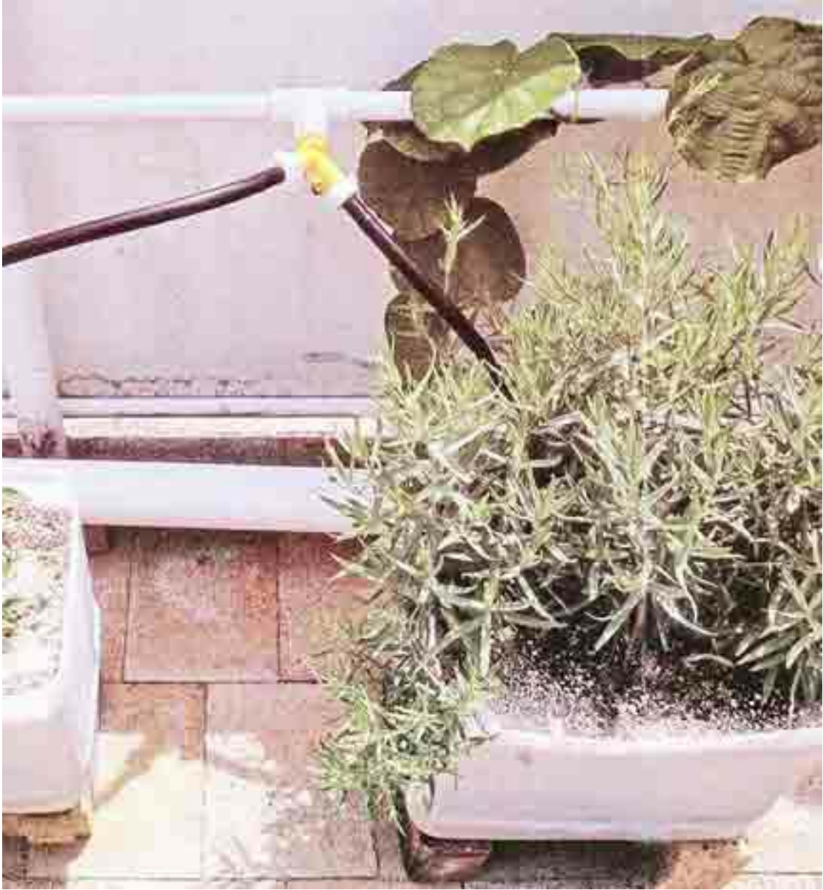
Feeder lines run from the main nutrient flow pipe running along this wall to a number of aggregate filled containers. The plastic drainage return pipe can be seen at the base of the wall.
