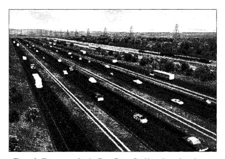
**Figure 2.** The concept for the Trans-Texas Corridor, shown here in an artist's rendering, calls for separate lanes for cars and trucks; rail with separate lines for passenger, high-speed freight, and commuter traffic; and a utility zone.
