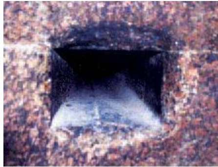
Entrance to the southern shaft from the Queen's Chamber, which was first explored in March 1993 by Rudolph Gantenbrink's robot. (Photographs by J. Douglas Kenyon)
