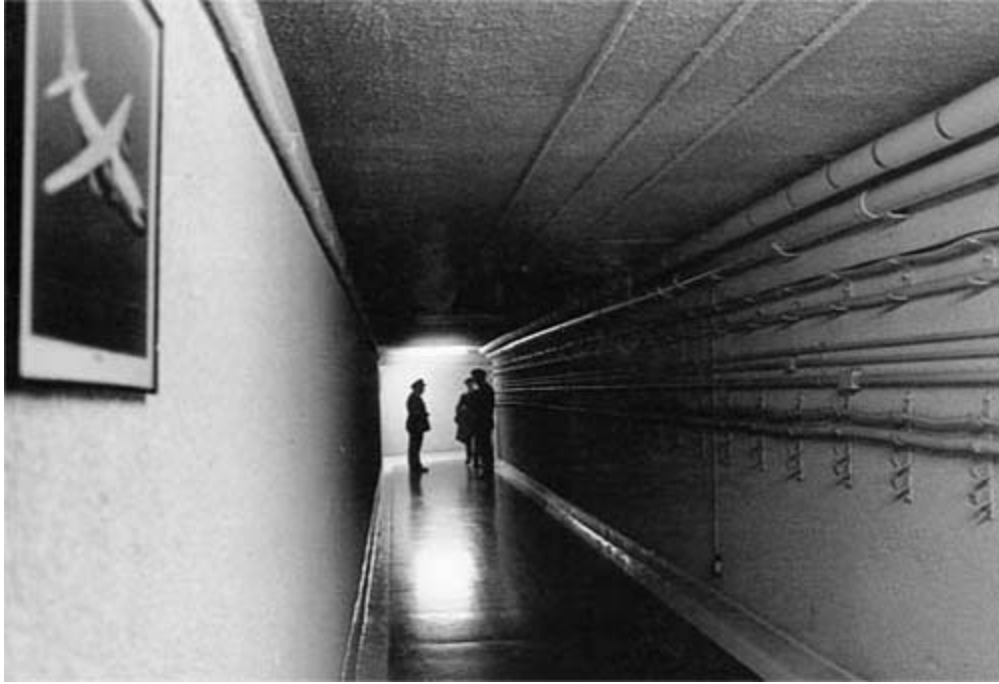
Bawdsey underground facility known as 'The Hole' (1974) courtesy Gordon Kinsey
