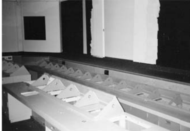
The primary control room showing the computer fittings and nuclear-proof walls, RAF Bentwaters (1999) © Georgina Bruni
