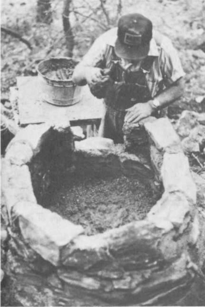
PLATE 434 When the walls were up about a foot above the bedstone, Buck removed the copper still and placed a 3"-thick layer of red clay on top of the bedstone to insure that no flames ever hit the bottom of the still and burned a hole in it. Then he proceeded with the next round of rocks, leaving an 11 1/2" hole in front for the scuttle hole or smoke vent.
