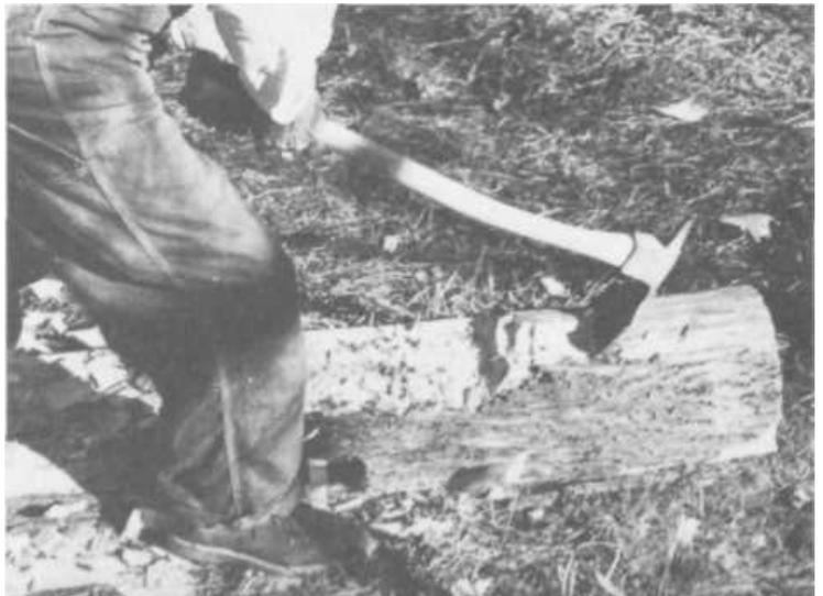
The adze was extremely sharp. Millard proved this to us by shaving about an inch of hair off his arm. He said he had to sharpen it before each log or it wouldn't work properly. Even with sharp tools, it is still hard work.
