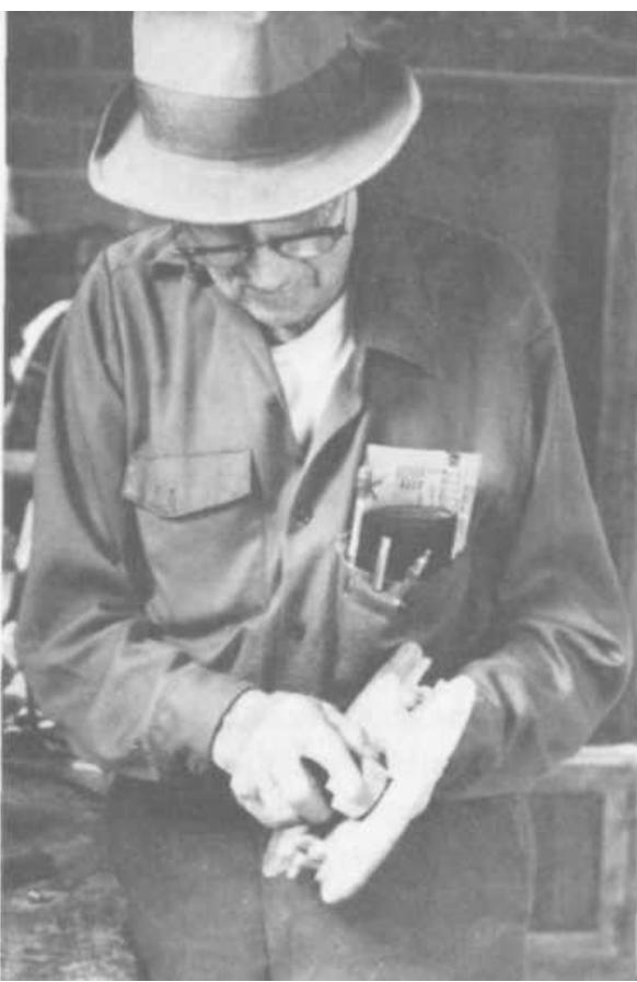
PLATE 113 With the plane, Harley shapes out the top and the back of the fiddle until they are about 1/8" thick.
