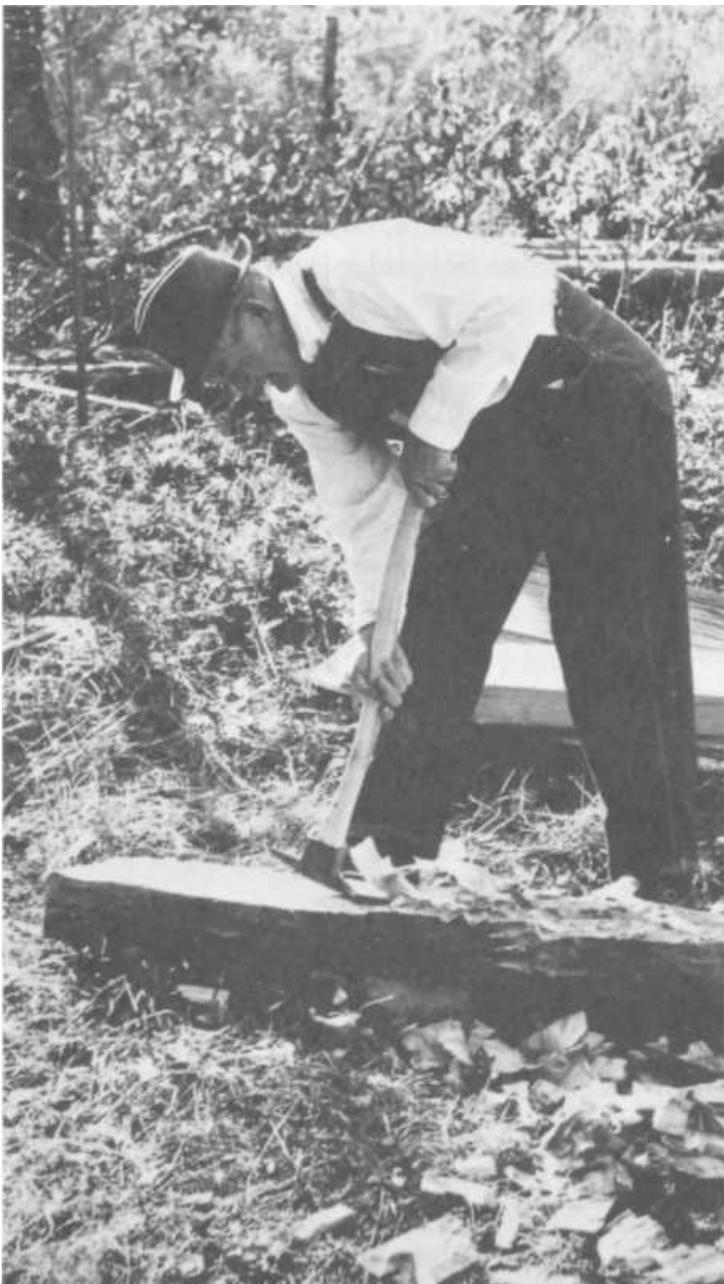
PLATE 408 Now, working backward, sometimes standing beside the log and sometimes straddling it, he goes over the rough-hewn side once again with smaller strokes to take off another 2" (thus getting the beam down to the thickness he wants) and smooth the side.
