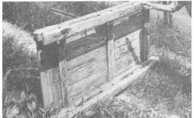
PLATES 184-187 (Variation #1) This sled, made by Tedra years ago, displays some notable differences from the one he made for our article. Both the runners and the half soles are in two pieces, the cross-pieces on top of the sills are inset, the front of the sills extends to the runners and are bolted to them, and the standards run beside the blocks rather than through them.
