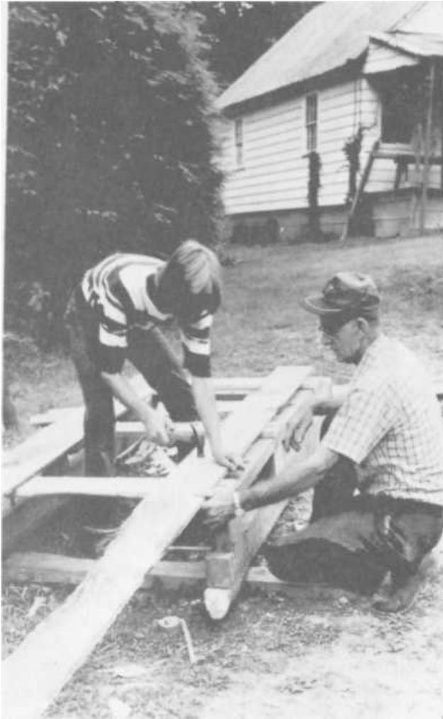
PLATE 182 After the other half sole is set the sled is righted and an oak floor is added. With the standards replaced, it's ready to use. Some farmers also make a long wood box with high sides that will fit down between the standards and rest on the floor. This is set on the sled when hauling small rocks, corn, and the like, and is removed when not needed.
