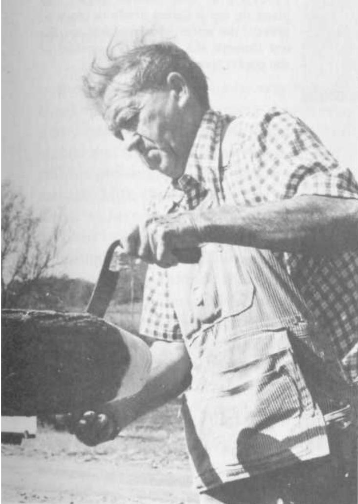
PLATE 312 When the pipe is drilled, he uses a drawknife to taper one end.
