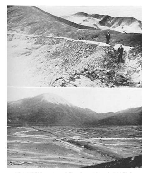
FIG. 79. The ancient civilizations of Peru had skilled engineers. In the upper view is seen one of the ancient aqueducts still intact for thirty-five miles which modern scientists estimate was capable of delivering sixty million cubic feet of water per day. They had no hardened tools or blasting powder, yet they cut this channel through boulders and rocks. Below is seen a valley covering thousands of acres once made fertile by irrigation but now an arid desert.
