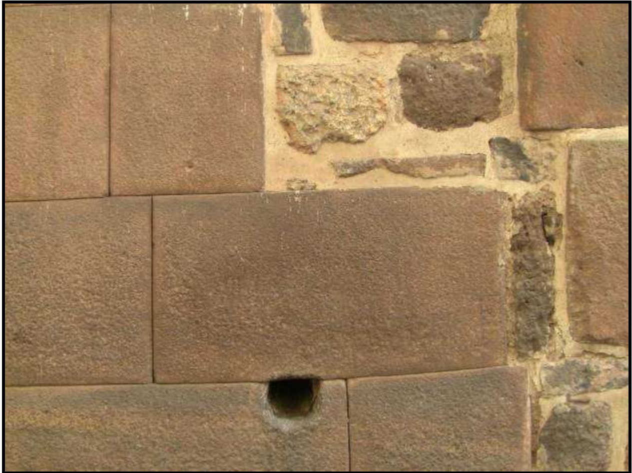
Proposed Inca stone work and later Spanish “repairs” using mortar
