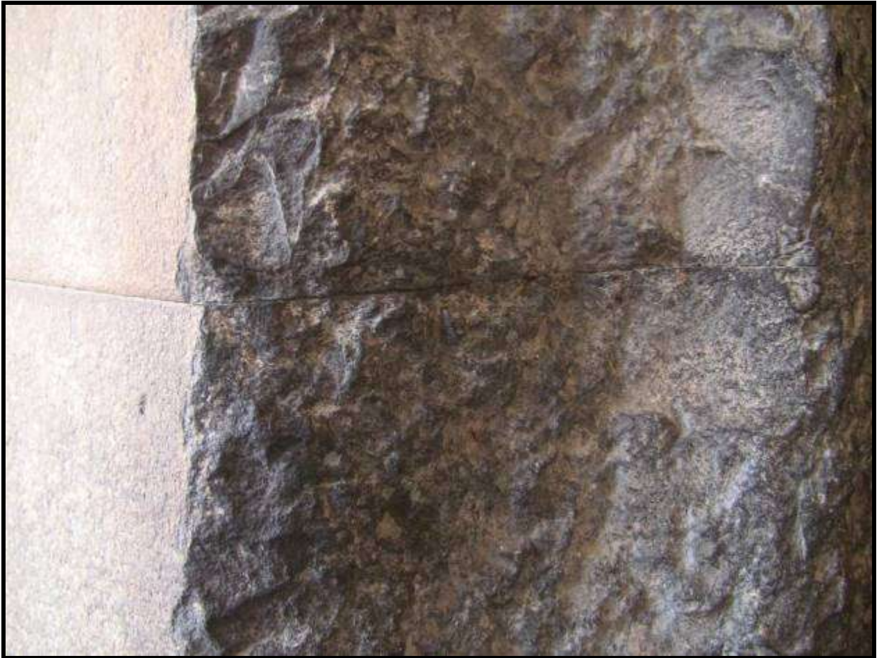
Broken wall section on the right side of the Temple of the Moon
