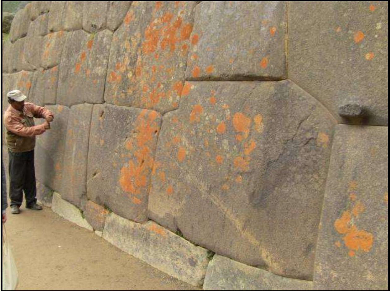
Polygonal wall below the Temple of the Sun at Ollantaytambo
