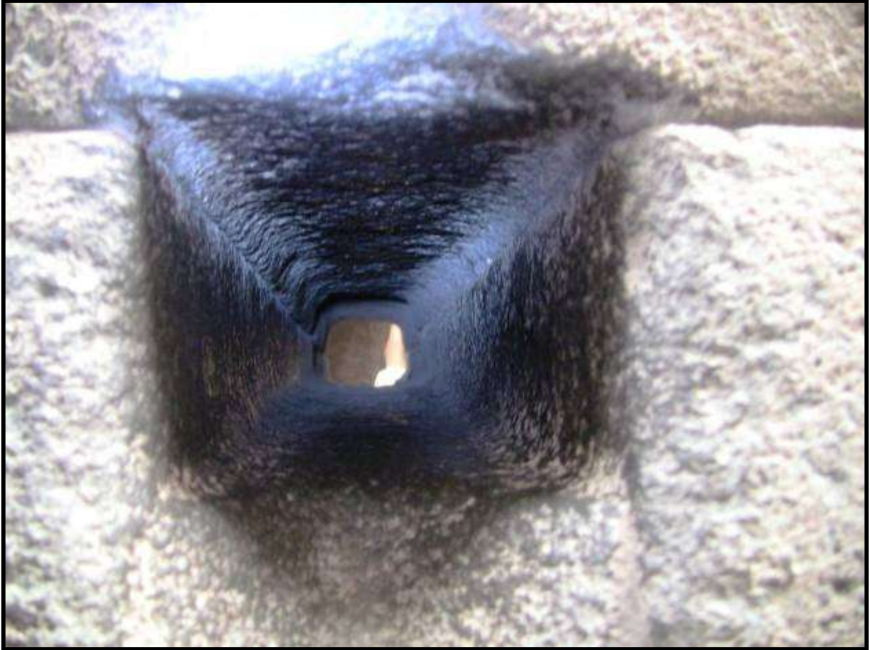
The incredible joinery goes right through the wall, more than a meter thick
