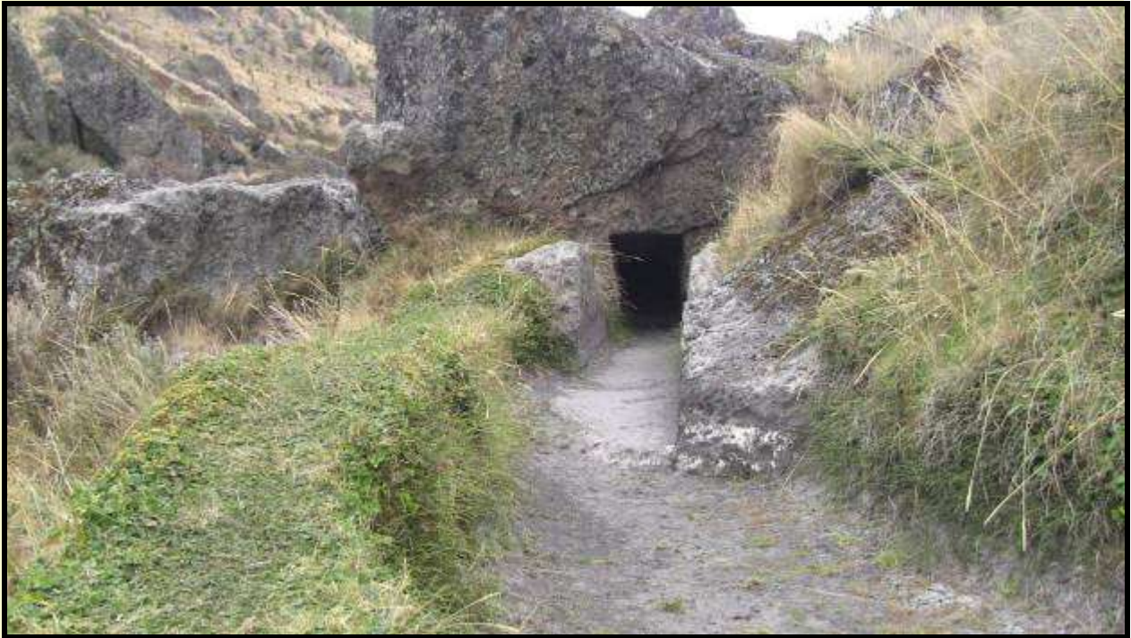
The aqueduct goes straight through this rock outcrop
