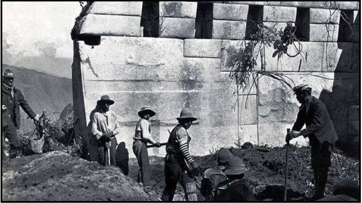
Early excavations of the “three sided structure”
