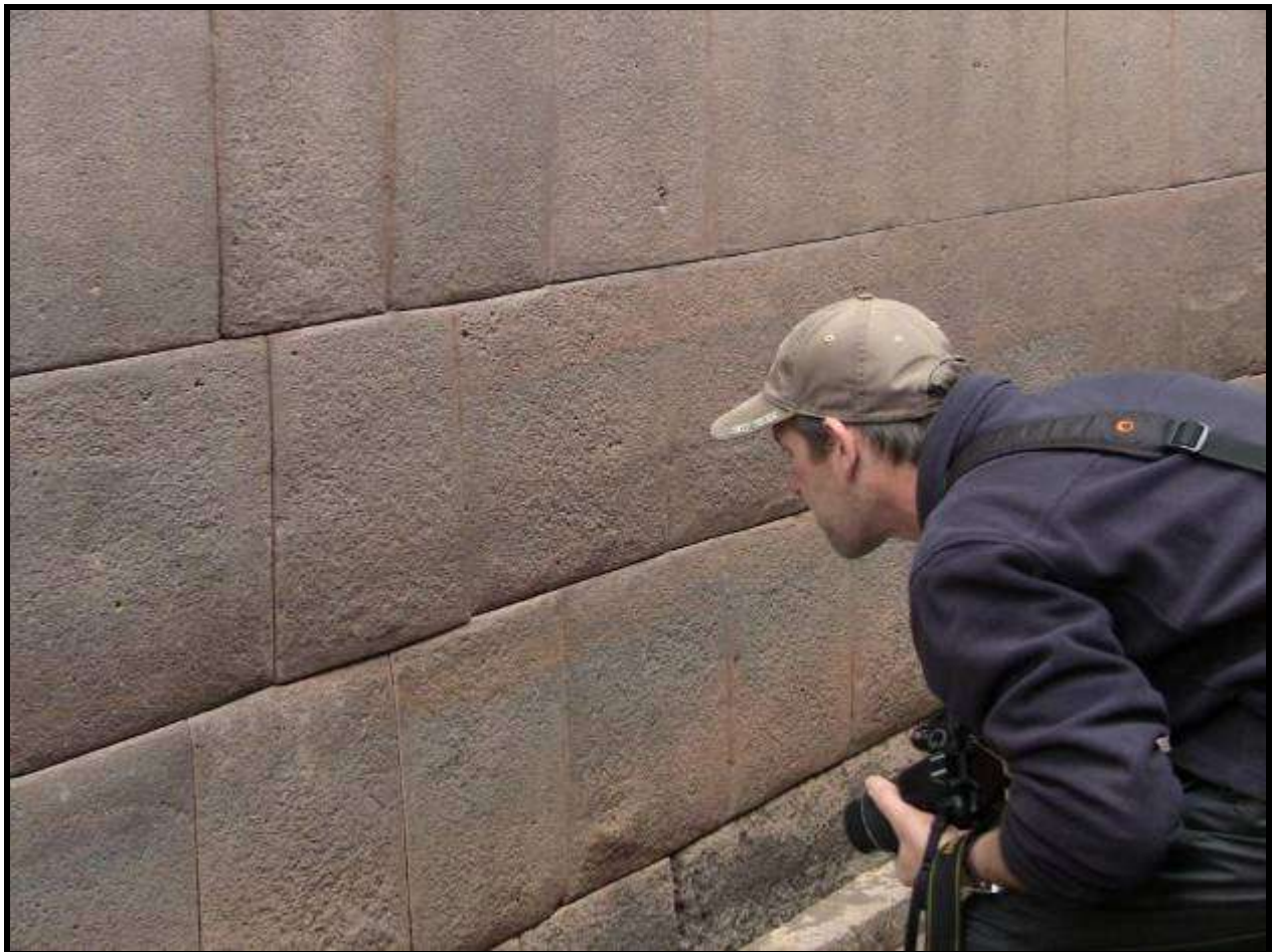
Engineer Dan inspecting the tight stone fit of the exterior wall of the Coricancha
