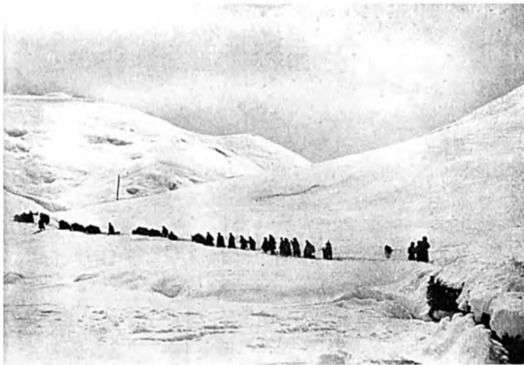
Men and yaks clearing the road to the Chumbi valley under deep snow.
