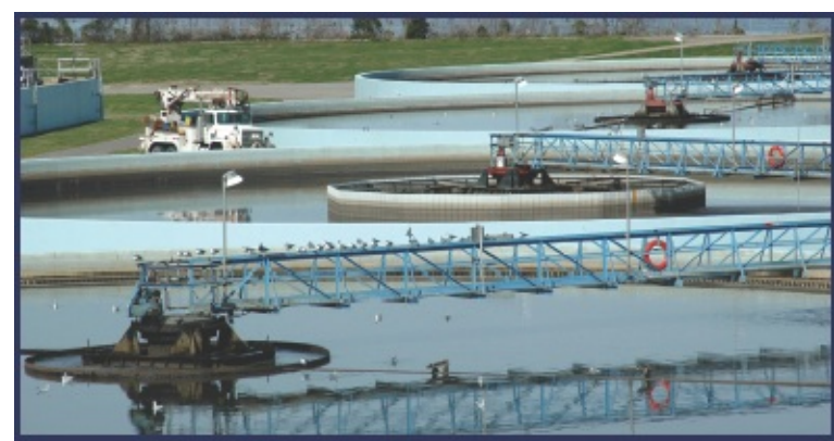
Water treatment facility (photo by FEMA/Manny Broussard)
