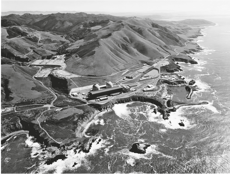
Diablo Canyon Power Plant in central California. (Courtesy of Pacific Gas and Electric Company)
