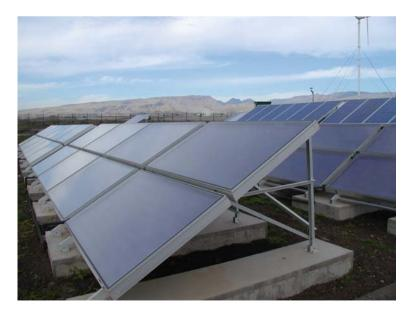
Fig. 10.4 The solar collector system of the 1 m<sup>3</sup>/day MD plant
