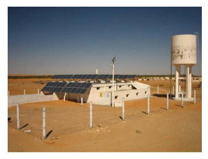
Fig. 10.5 The building housing the RO system, the PV and the water storage tank of the PV/RO system in Tunisia
