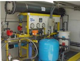
Fig. 10.7 The ITC wind/RO system in the Canary Islands
