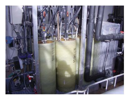
Fig. 7.14 Desalination unit with five MD modules and heat exchanger (on the right)
