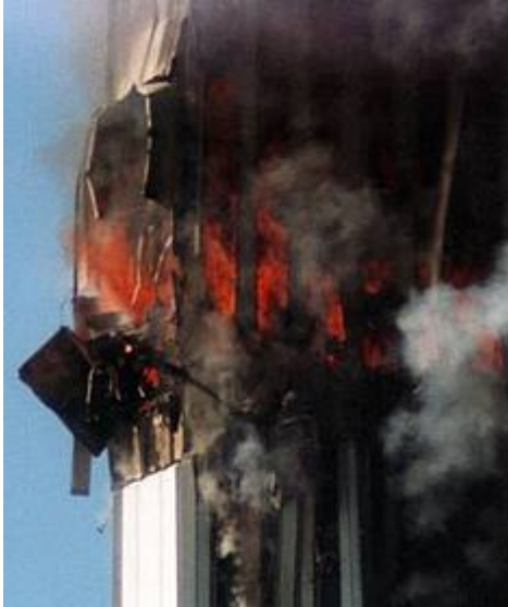
Exit hole in NE corner of WTC2
