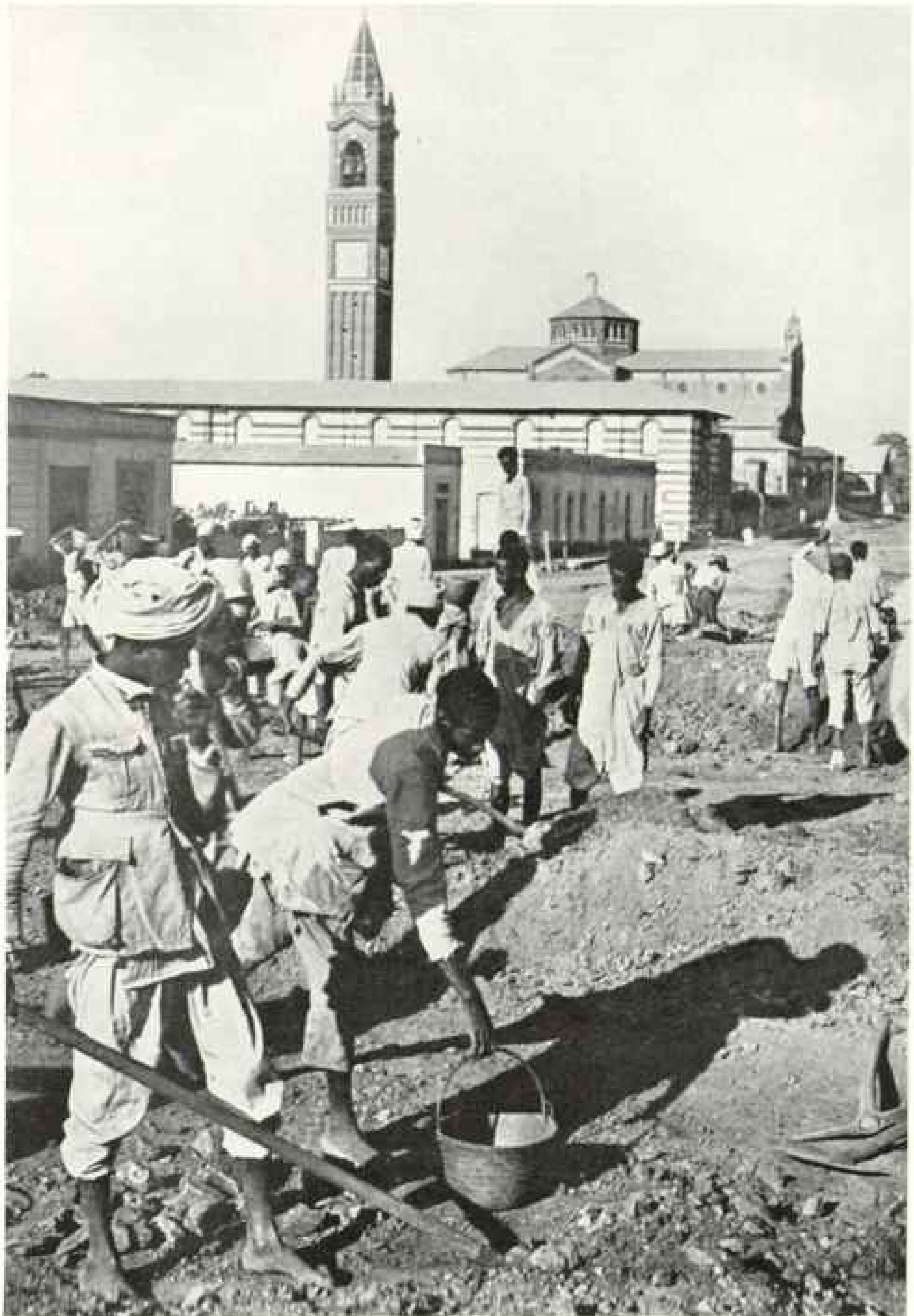
IN HONOR OF IL DUCE, MUSSOLINI STREET IS BEING PAVED AND WIDENED
