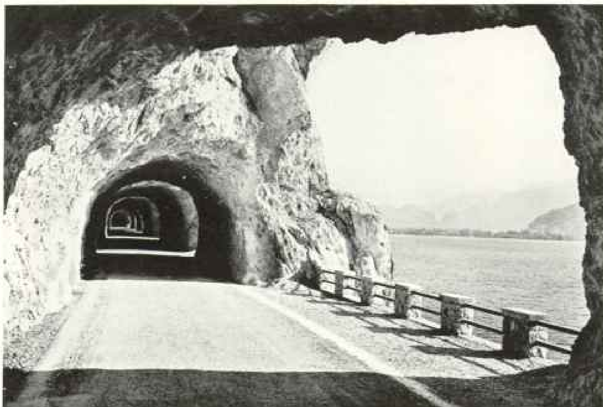
THE WAY OF THE TITANS BORES THROUGH SOLID ROCK ALONG GARDA'S EDGE
