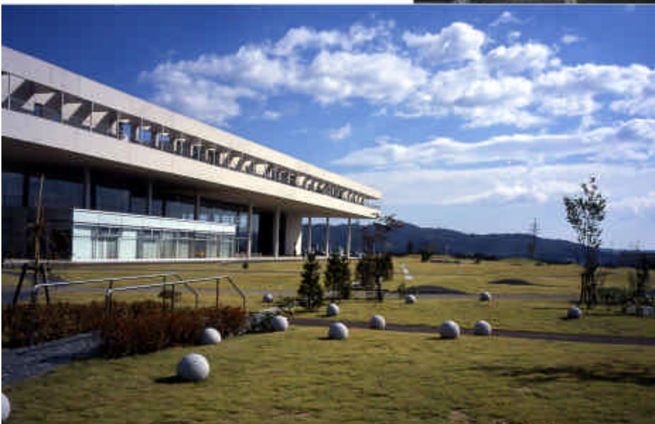
The Katta public general hospital has many sustainable factors such as passive energy saving, cogeneration system, natural lightings and ventilation by natural draft. It is also functional even if the elevator stops due to the earthquake because this is low layer construction. The healing garden designed based on the advice from the hospital workers function as a part of the treatment program for the patients:
