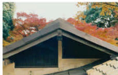
Air in the house flows out to the attic through the vent established on the ceiling or RANMA (transom window).
