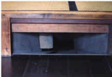
Cool tube is an airway carrying the air from west side of the building to the living room. The heated air cools down by the earth temperature. The gateway of the tube is implanted in the step of the Tatami.
