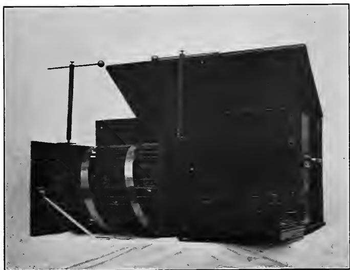
PLATE III. — Oscillation Transformer and Glass for Condenser of 12" Coil.
