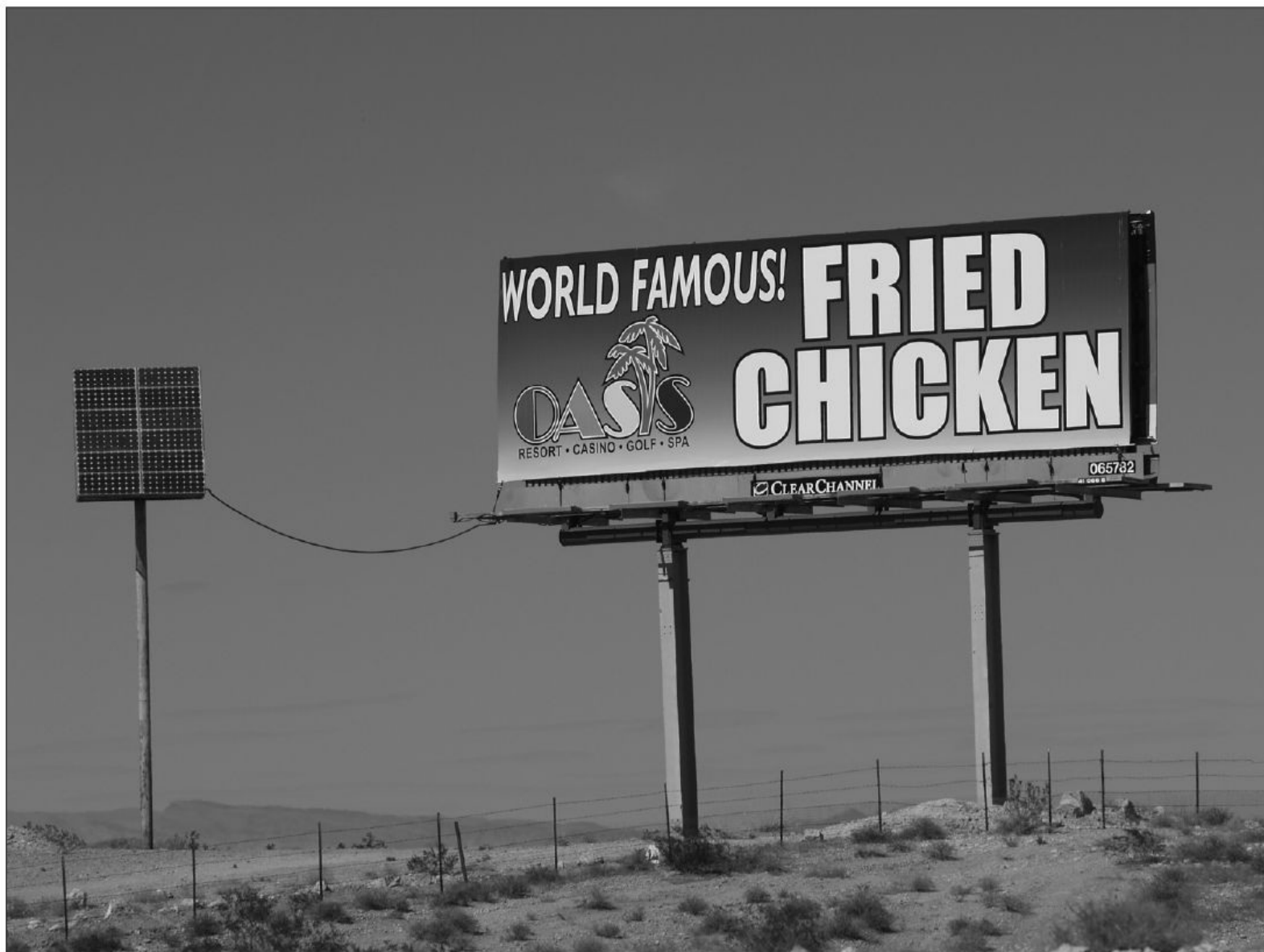
Pole-mounted panels powering billboard lights.
