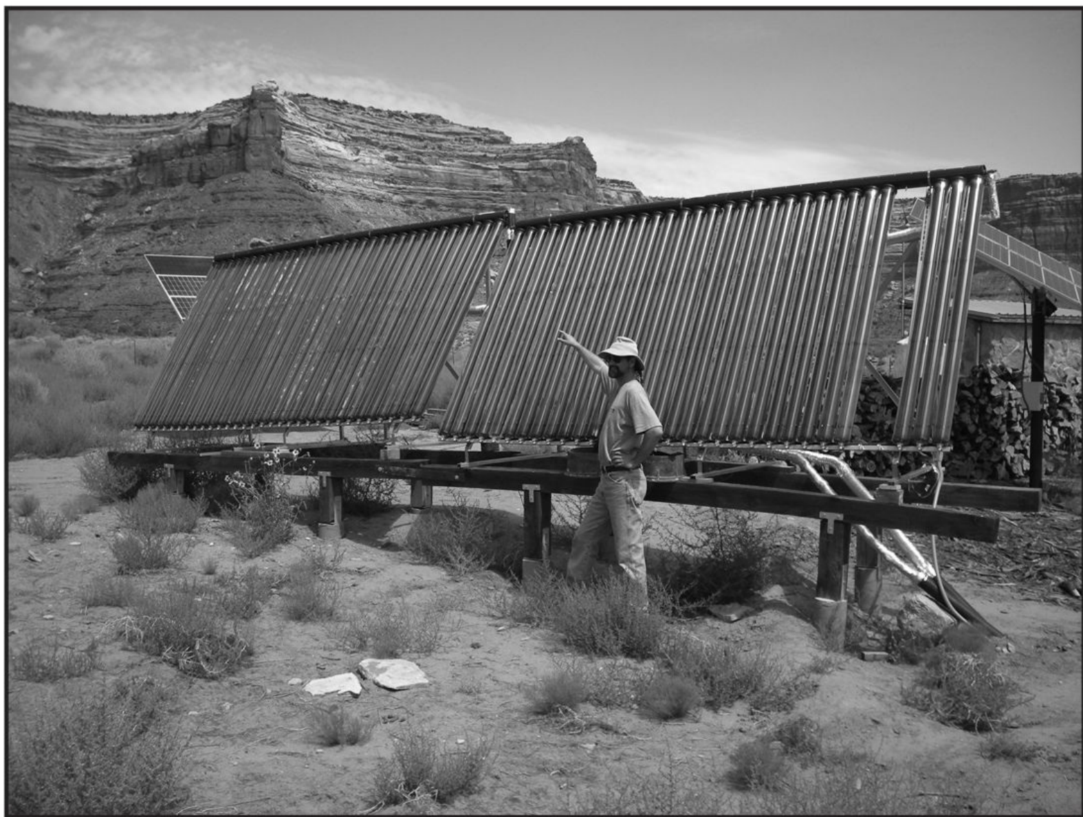
Evacuated tubes: This evacuated tube system at Valley of the Gods B&B provides hot water for the owners and four guest rooms.
