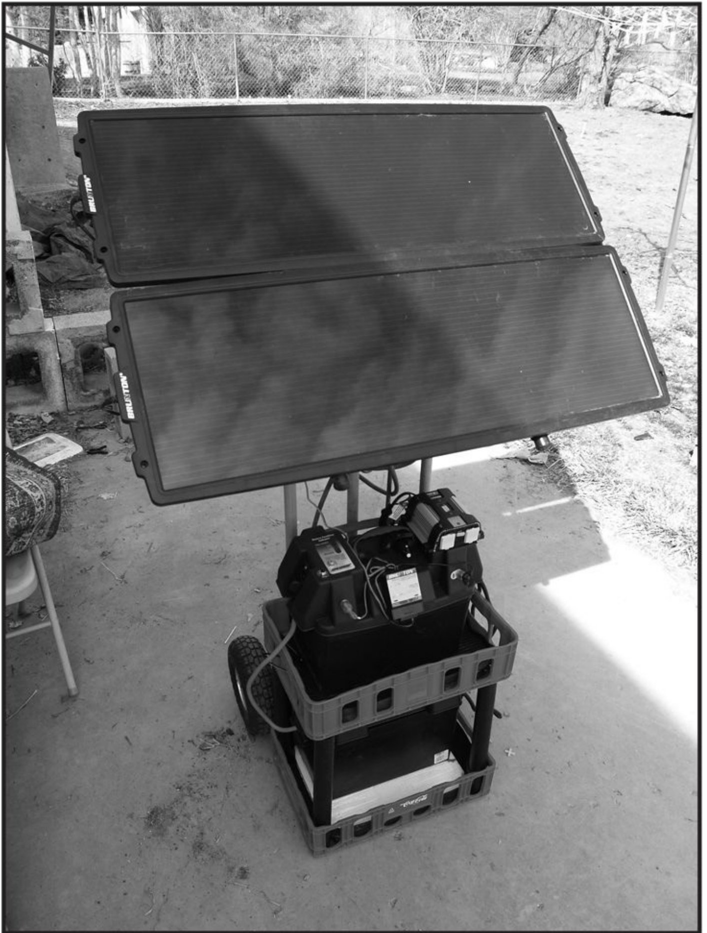
Portable emergency 12V system with two batteries in parallel and two, 1-amp 15-volt panels in parallel, making a 12V, 30W system. In this parallel PV panel array, all the red wires (+) are
