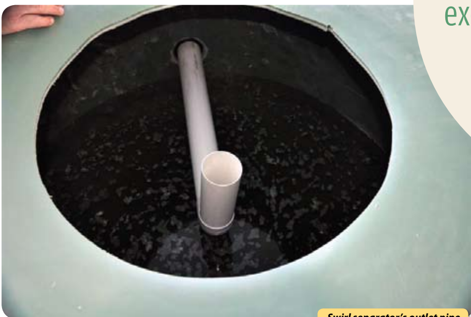
Swirl separator's outlet pipe
