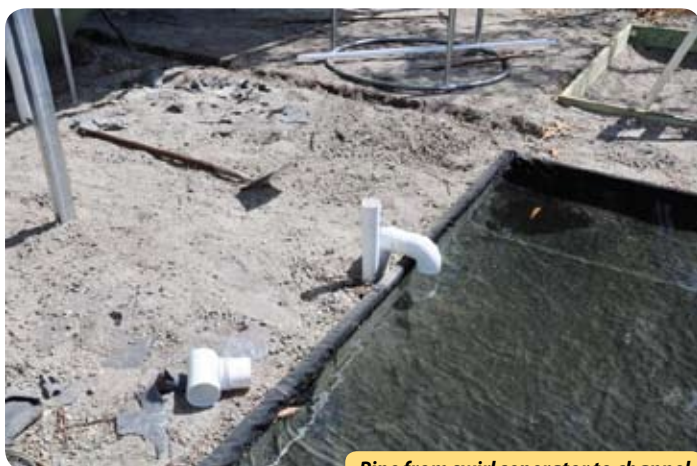
Pipe from swirl separator to channel
