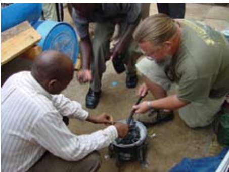
Using charcoal in a "Jiko" (pronounced gee-ko) to gently heat the suction tube so we can bend it.
