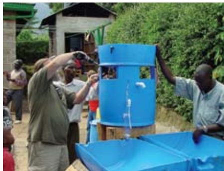
Installing the top raft tank onto the flood tank of the system. The growbeds and fish tank are already almost completed.
