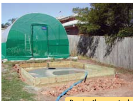
Burying the sump tank
