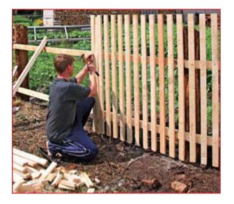
A picket fence is constructed by nailing two or more long boards to posts, and then nailing narrow vertical boards to the horizontal ones.
