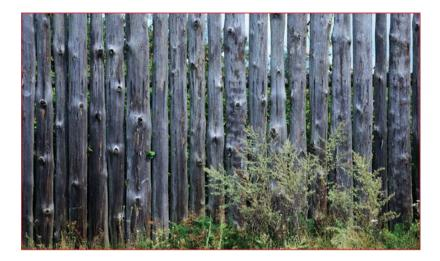
. A very simple fence can be made by driving small tree trunks or branches into the ground in a tight row.
