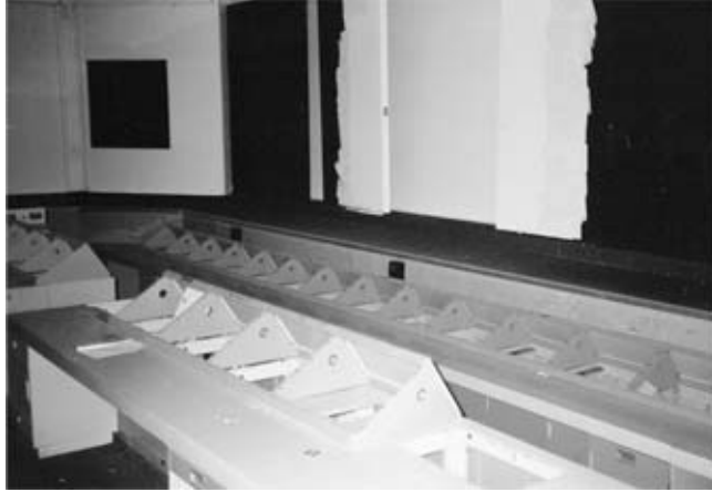
The primary control room showing the computer fittings and nuclear-proof walls, RAF Bentwaters (1999)
