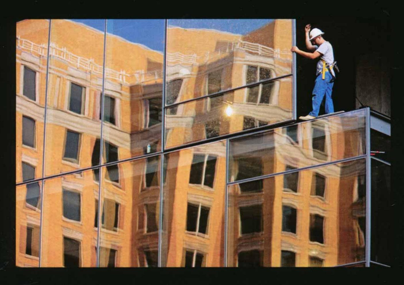
A worker in Washington, D.C., installs a triple-glazed window in a structure designed to meet strict "green building" standards. Advanced lighting, heating and cooling, and water systems, and a green roof contribute to a small carbon footprint, and can reduce energy costs by up to 75 percent. But many firms hesitate to invest in efficiency if up-front costs seem too high or payback times too long.
