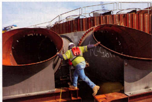
Pump discharge pipes at London Avenue gates (4)
