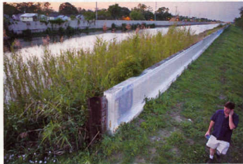
A floodwall gap on the Orleans Avenue Canal (3)
