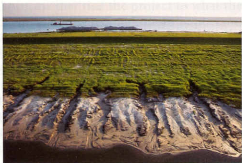
Erosion on the MRGO levees (8)
