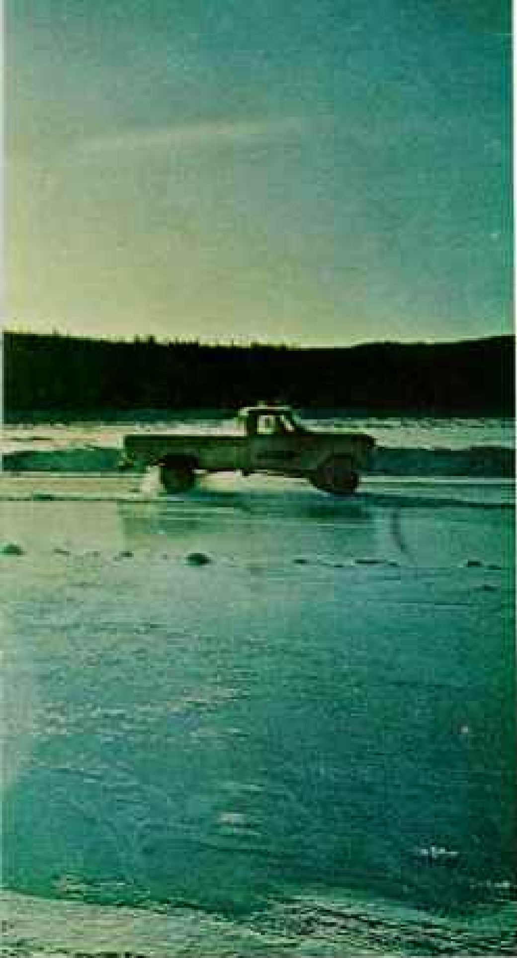
The glassy span slowly spreads from bank to bank (right), a link in the road carved in 1968-69 between Fairbanks and the North Slope. Spring revealed the price of careless construction: Uncovered permafrost along the bulldozed route thawed into an impassable trench.
