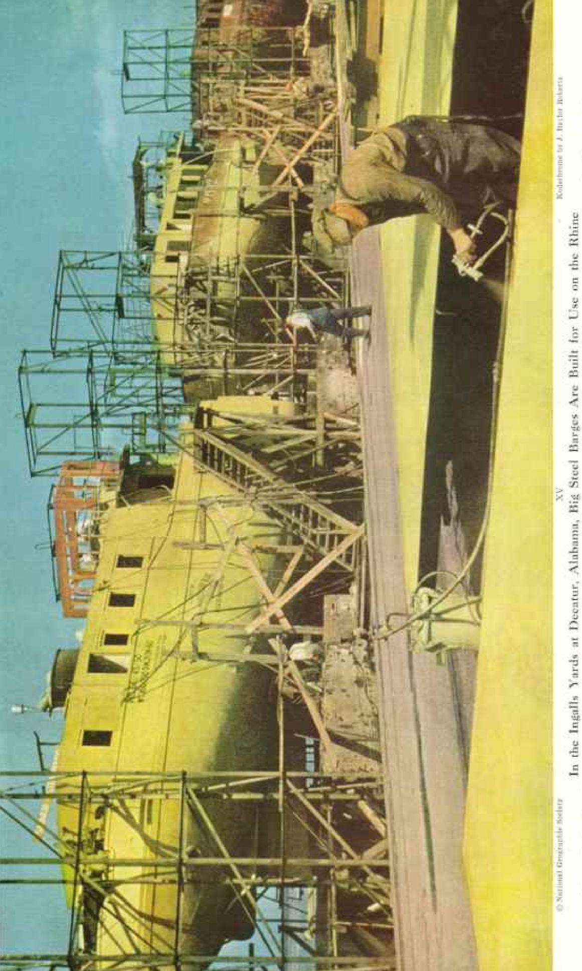
France bought 25 of the self-propelled craft. They are shipped down the Tennessee and Missisphi to New Orleans, thence by sea to Rotterdam for amembly. In the Ingalls Yards at Decatur, Alabama, Big Steel Barges Are Built for Use on the Rhine
