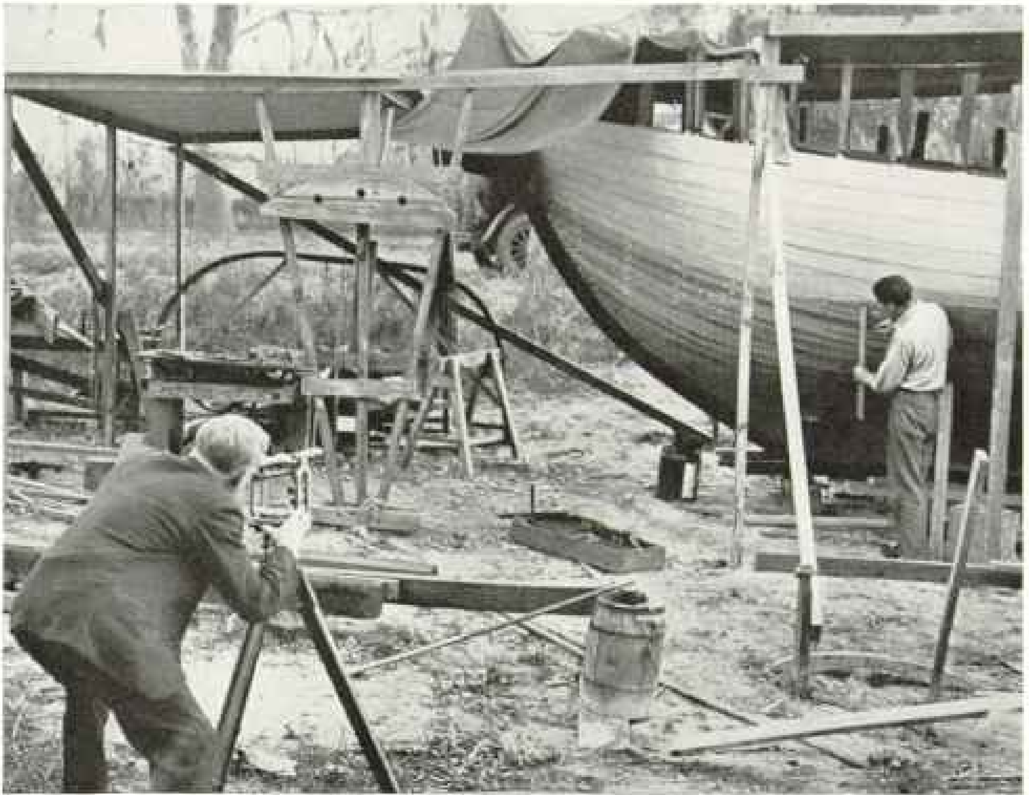
TRANSIT AND GAUGE CHART A STRAIGHT WATERLINE FOR "IGDRASIL"
