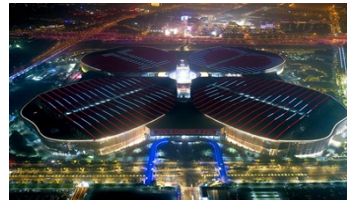
Night view of National Exhibition and Convention Center (Shanghai)
