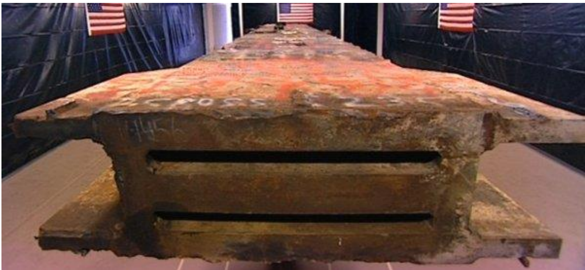
This image from the documentary Up From Zero shows the base of a core column, whose dimensions, minus the four flanges, are apparently 52 by 22 inches, with walls at least 5 inches thick.
