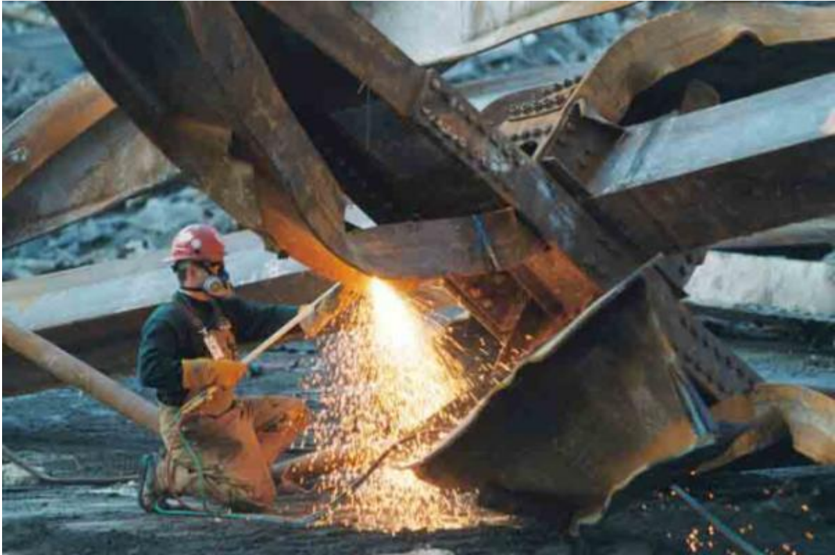
This photograph from Ground Zero is apparently of one of the smaller core columns connected to a set of I-beams.
